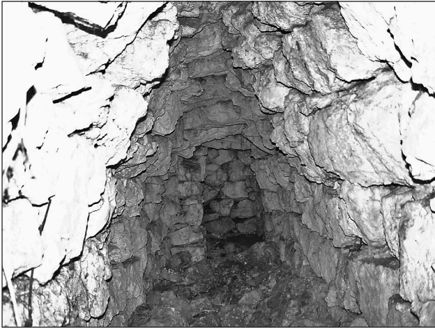
Figure 4. Photo of the entry passage of cave 1 showing details of construction. Note the portion of the wall extending in passage (left, rear) that may have acted as a light baffle (photograph by Alezandra Brady).
