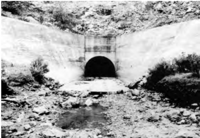
Entrance to 5 kilometer long tunnel.
