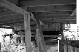
Left: After a decade on the original posts, the warping and bending are obvious. The outside corners the house had settled over 25 centimeters. Below: The fieldhouse sitting on new block foundation walls, Spring 2009.
