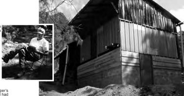
May 2009: Only some flashing remains before the new room will be dried in. A retractable porch will extend at the 2nd floor level when the job is finished.
