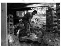
Hired help: Mario demolishes the large rock where the walls will stand. Around him is the 4X4 cribbing used to jack up the house.
