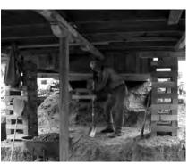
Ediger operating the excavator on the helper's day off. About 120 centimeters of material had to be excavated just to get to floor level on the high end. The bottom of the footer was another
