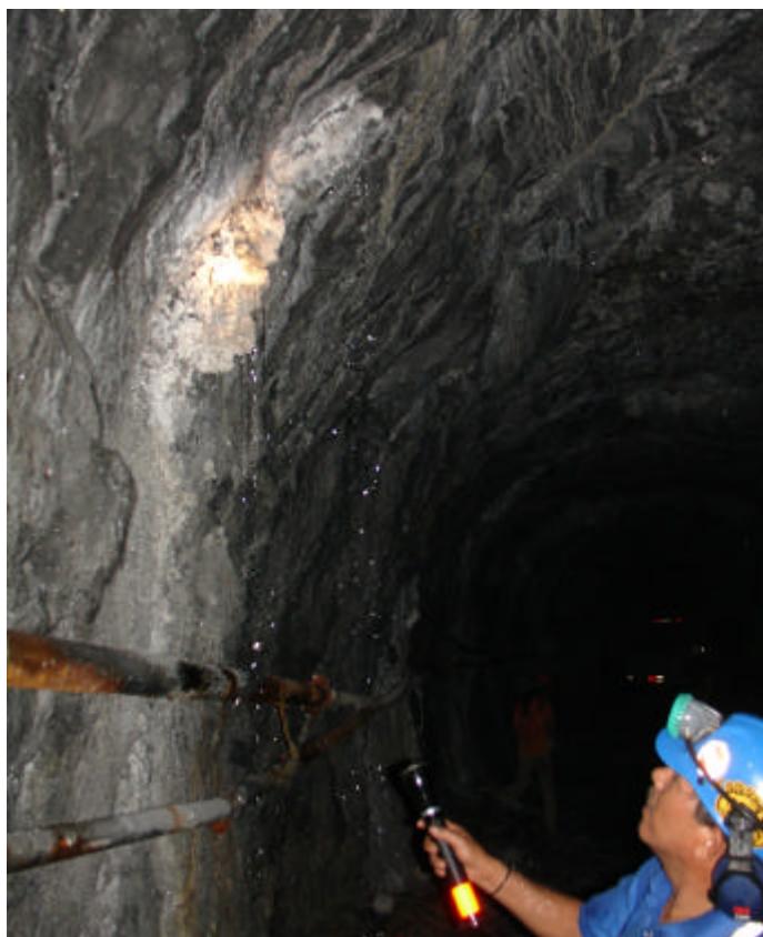
Fig. 1- Thermal water spilling out in the -590 gallery (photo La Venta and Speleoresearch & Films)
